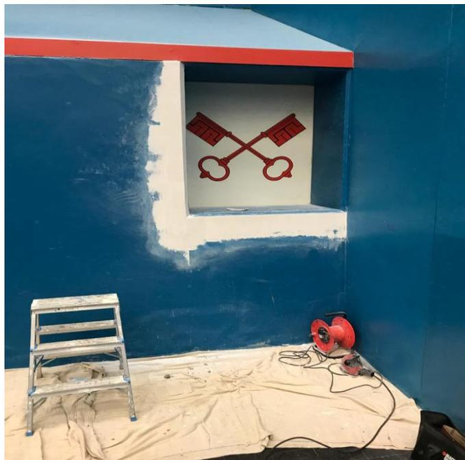
These include remodelling the look of the grille, eliminating the wooden frame that has not proven to be a satisfactory arrangement. The pounding it receives dislodges it from the plaster, which then breaks up under impact, and things have just got worse and worse. But no more, we hope.
